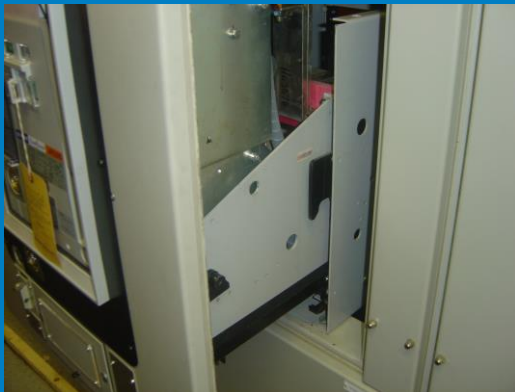
Transplanted ACB in original rolling shell
