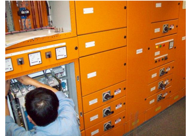
Working process at Jimblebar Mine
